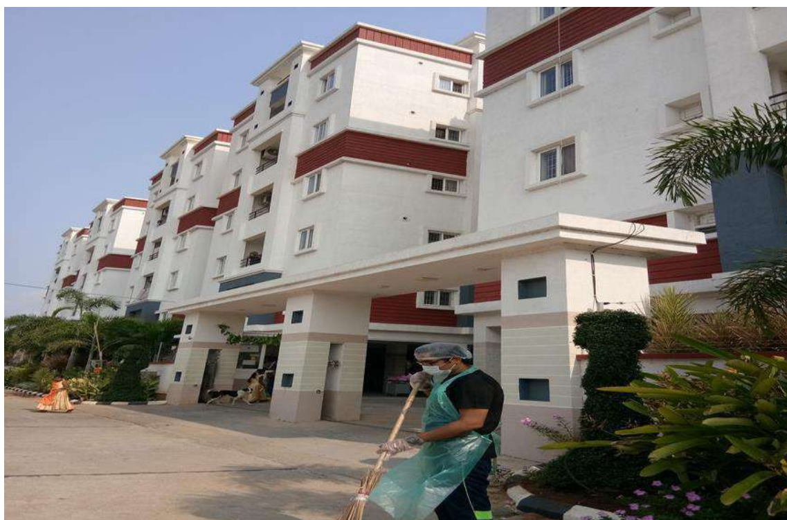
Temporary hostel facilities at SLV Anjani heights, Gannavaram
